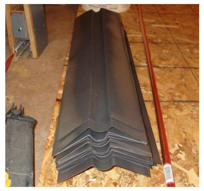
Once that was done, I attached a narrower piece of flashing to the back of each fin, using self-tapping sheet metal screws down one side only, with silicone in between for slightly better heat transfer (yeah I know, silicone is not a great conductor, but as Gary points out, it's a lot more conductive than air, so it's better than nothing). To attach them to the copper pipe, I can just slide it on and screw down the other side.
