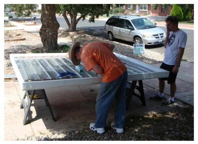
And then some corrugated polycarbonate glazing on the front, attached with short hex-head screws with rubber gaskets. I drilled the holes in the poly considerably larger than the screws, since it'll want to expand and contract (and I don't want it to crack). Of course, liberal use of silicone here too.
