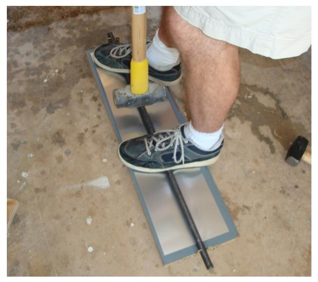
Aluminum flashing is pretty springy, so they don't keep the shape very well, but it's a pretty good start at having the wrap-around profile I'm looking for. In order to mitigate possible galvanic corrosion between the aluminum and copper, I painted the inside grooves black using high-temperature barbecue paint. It doesn't need to be black, but I was planning to use this paint on the rest of the fins anyway.
