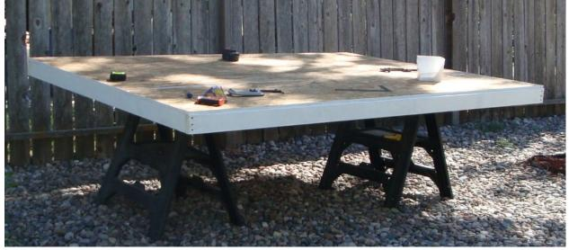
the box. I made mine using 2x4 lumber and 1/2" plywood. It's 8 feet wide by 6 feet high:
